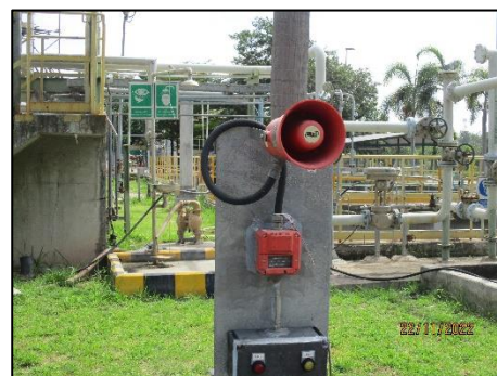
Fire Alarm Manual Station
