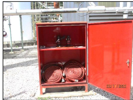
Fire Hose Box and Nozzle
