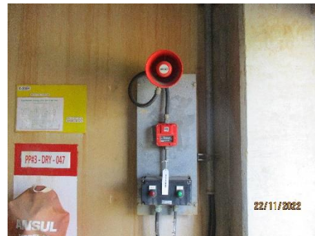
Fire Alarm Manual Station
